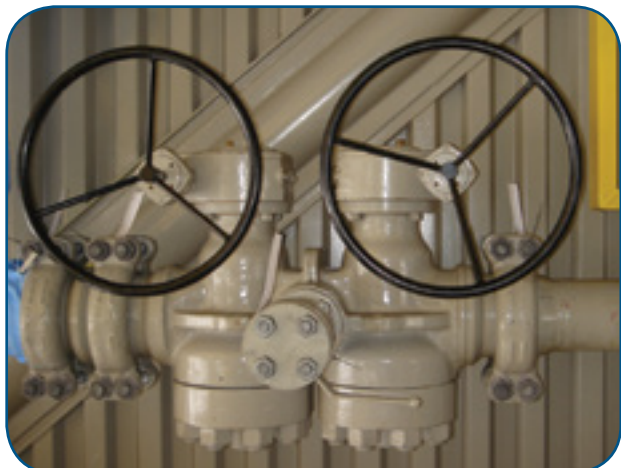
The valves illustrated are 6" class 2500 with hub ends, in carbon steel, manually operated. criteria for selection: bubble tight isolation and compact design.
