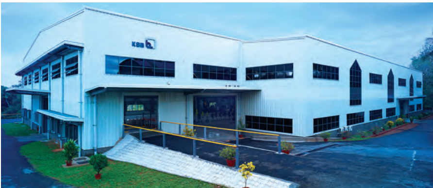
Exterior view of large valve manufacturing plant of KSB MIL, Kerala, India
